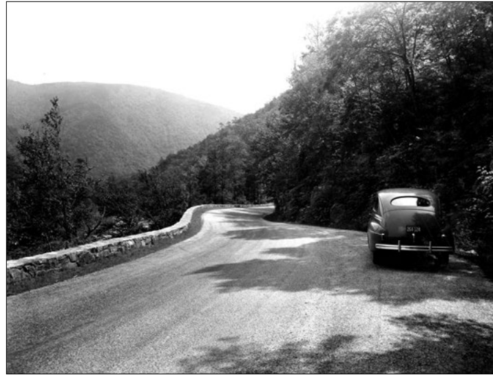
State highway built in 1939 through Goshen Pass: a rare instance of a road as roads ought to be built
